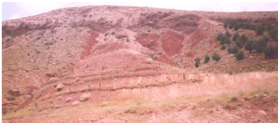
Fig (8): Cultivated stages along the Gercus slopes to block the rolled fallen rocks.
