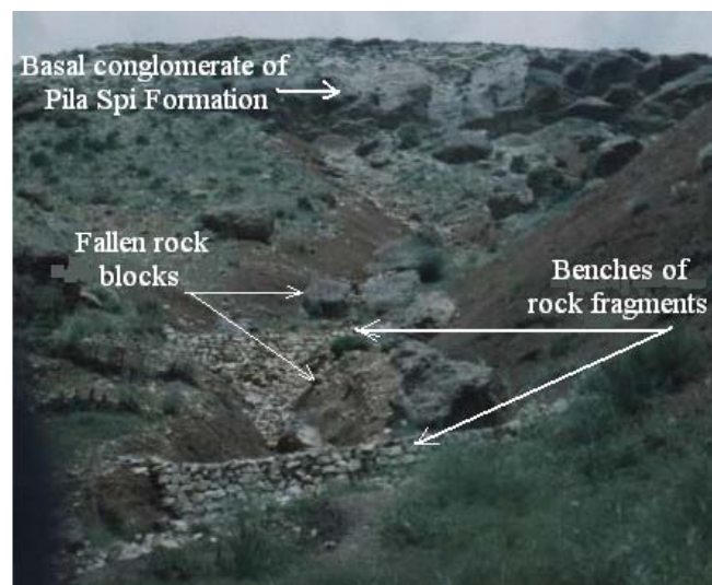
Fig (6): Rocky stages and benches to restrain and prevent the fallen rocks from reaching the slope's toe.
